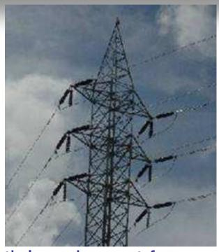
Electrical insulators is one of the essential equipment for the electricity's transmission and distribution systems. It can prevent the electricity leaks from the conductor to the ground which would cause the short circuit and cause the unplanned electricity outage. Another main duty of insulators is to hold and suspend the electrical conductor in the air.
