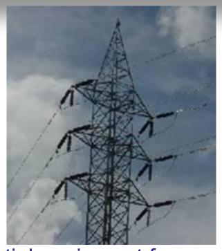
Electrical insulators is one of the essential equipment for the electricity's transmission and distribution systems. It can prevent the electricity leaks from the conductor to the ground which would cause the short circuit and cause the unplanned electricity outage. Another main duty of insulators is to hold and suspend the electrical conductor in the air.
